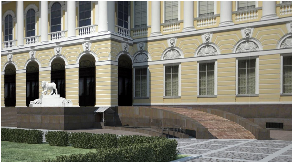
Figure 3 - The ramp and carriage entrance (AMS).
